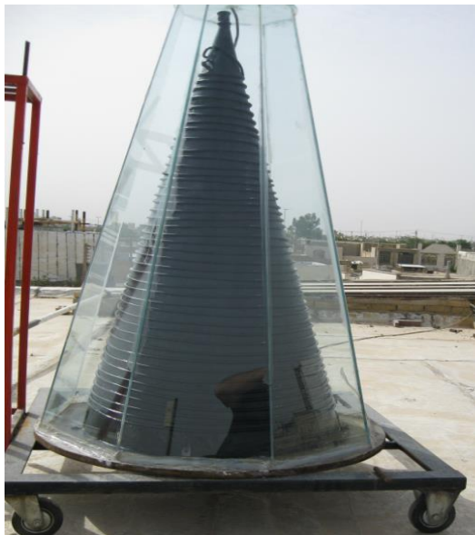
Fig. 2 Piping and cover install on a conical solar collector.
