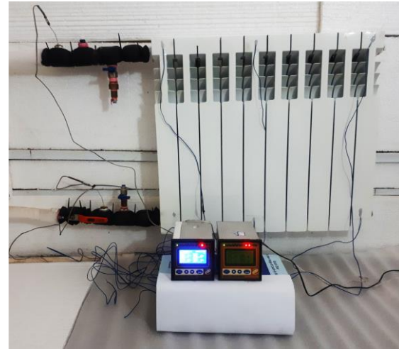
Fig. 5. The radiator and connections
